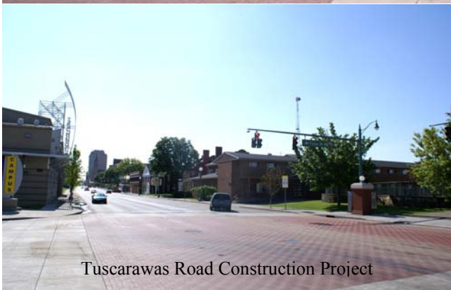
Tuscarawas Road Construction Project
